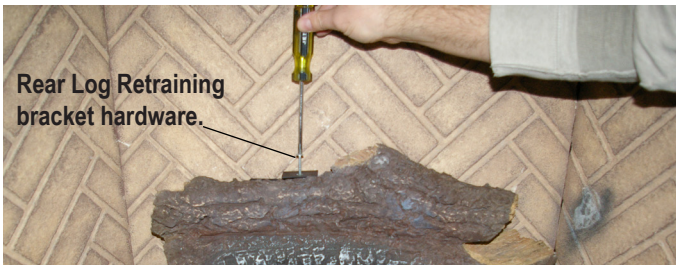
Figure 31b. Fastening Retaining bracket to Rear Log.
