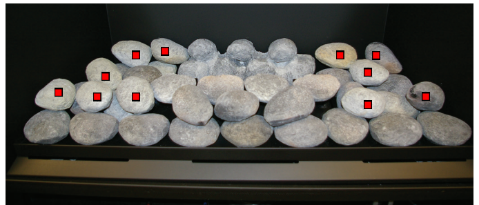
Figure 30g. Placement 11-faux ceramic rock "F", (as shown).
