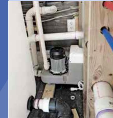
The Sanicom 1 drain pump showing the 1-inch discharge pipe running vertically to discharge the gray water from the washing machine into the blackwater tank. The washing machine will drain into the Sanicom 1 via a 2-inch inlet (on the left).
