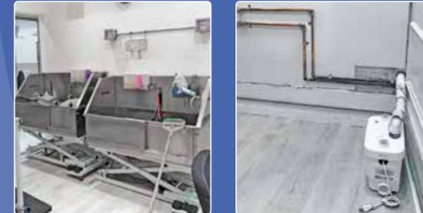
The two, 50-inch tubs used for daily grooming. The 1.5-inch rigid pipe connected to an existing PVC discharge pipe running to the building's sewage access.
