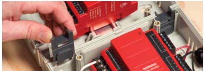
The convenient channel connectors allow you to easily add expansion zoning panels without running wires outside of the panels. This eliminates the risk of having wires exposed to the homeowner outside of the panel, and makes for a clean and organized installation.
