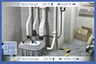
Discharge rate at 36' (2"): 26 gal/min (136 liters/min)
