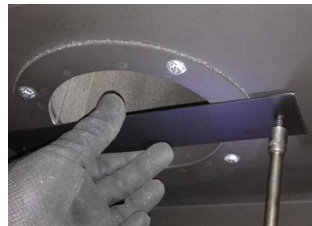
Figure 8.b.c Restrictor plate Installation
