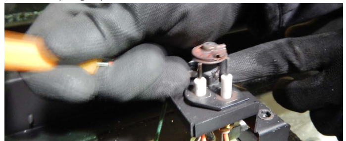
Figure 13.d Removing the spring clip
