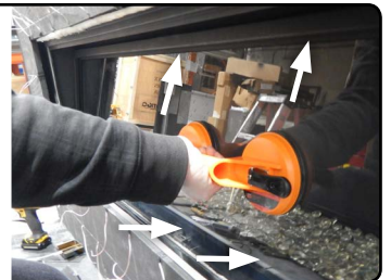
Figure 21.b Installing the door
