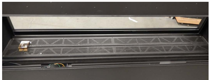
Figure 25.g. Insert pilot cover/door/screen
