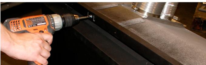
**Figure 3.3** Secure Slide plate
