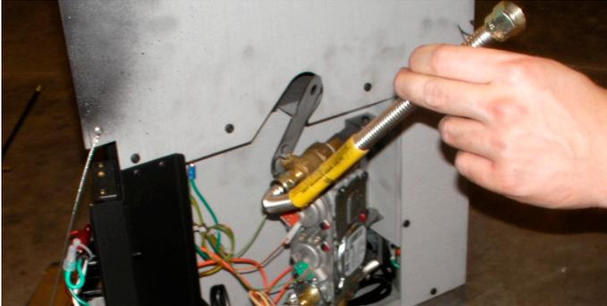
Figure 4.3 Converting the gas regulator on the valve
