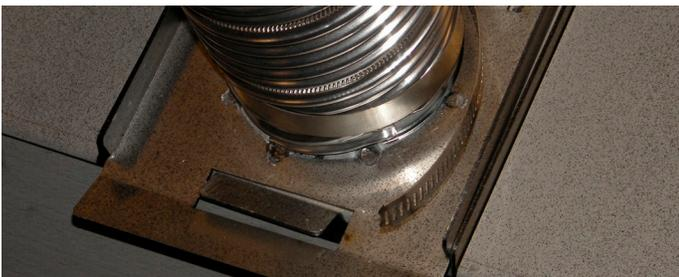
**Figure 3.2** Vent Slide plate
