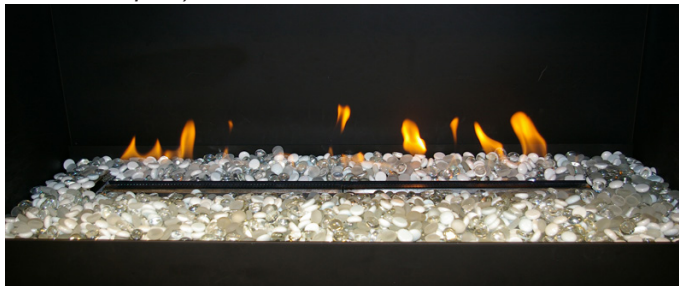
Figure 31a. Operating gas fireplace with firestones surrounding burner tray.
