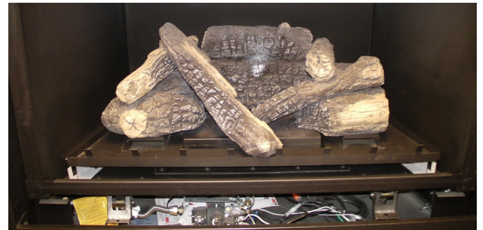
Figure 32a. Firebox with logs prior to ceramic fibre rock installation.
