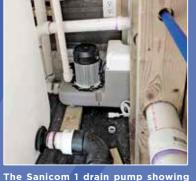
The Sanicom 1 drain pump showing the 1-inch discharge pipe running vertically to discharge the gray water from the washing machine into the blackwater tank. The washing machine will drain into the Sanicom 1 via a 2-inch inlet (on the left).
