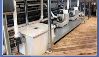
A 1-inch PVC drain line is connected to a three-bay sink and dishwasher situated to the right of the pump trio. This drain line first runs into a grease trap before connecting to one of the Sanicom 1 units.
