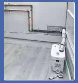
The two, 50-inch tubs used for daily grooming. The 1.5-inch rigid pipe connected to an existing PVC discharge pipe running to the building's sewage access.
