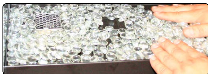
Figure 24. spreading out firestones
